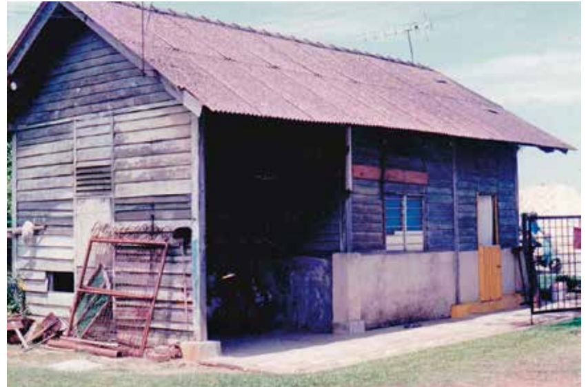
The car garage and the caretaker's house (1980s)
